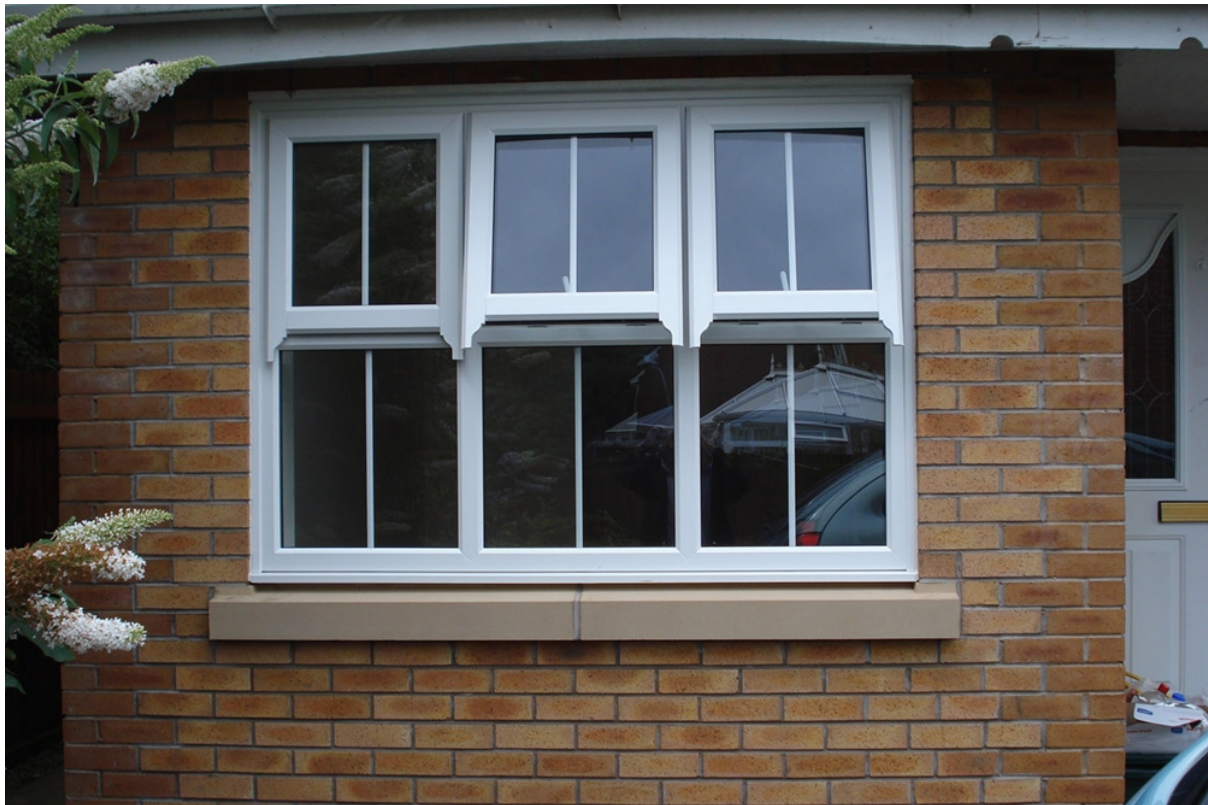
Example of a garage conversion where the former garage door was replaced by a window matching the house's style. Ensuring that a new front window aligns with existing windows and uses matching materials (brickwork, frame, and sill) helps maintain a harmonious appearance in the street scene.
